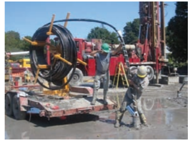
Inserting loop in bore hole on a commercial job.
